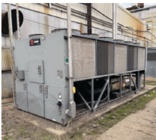
Trane Air-Cooled Series R Chiller
