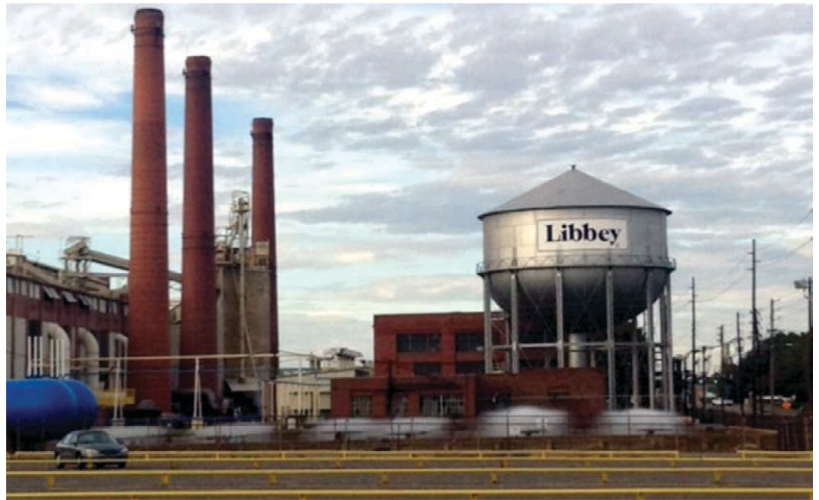
View of Libbey Glass Facility
